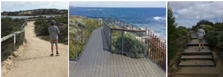
Figure 3.6 Walkways types including compacted limestone, boardwalks and boardwalks over dunes incorporating stairs.
