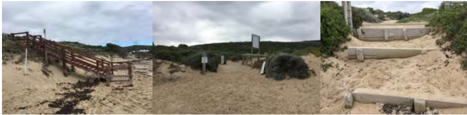
Figure 4.1 Beach Access Types including Timber Stairs (L), Retained Timber (C) and Sand Access (R).
