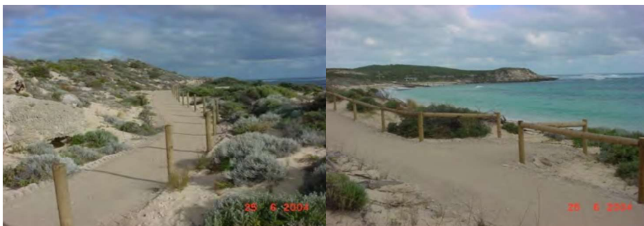
Figure 3.2 Coastal Walkway Stage 2 & 3 Constructed in 2004.
