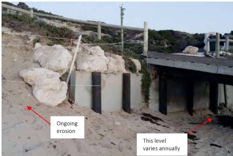
Figure 5.3 Gnarabup Boat Ramp Abutment
